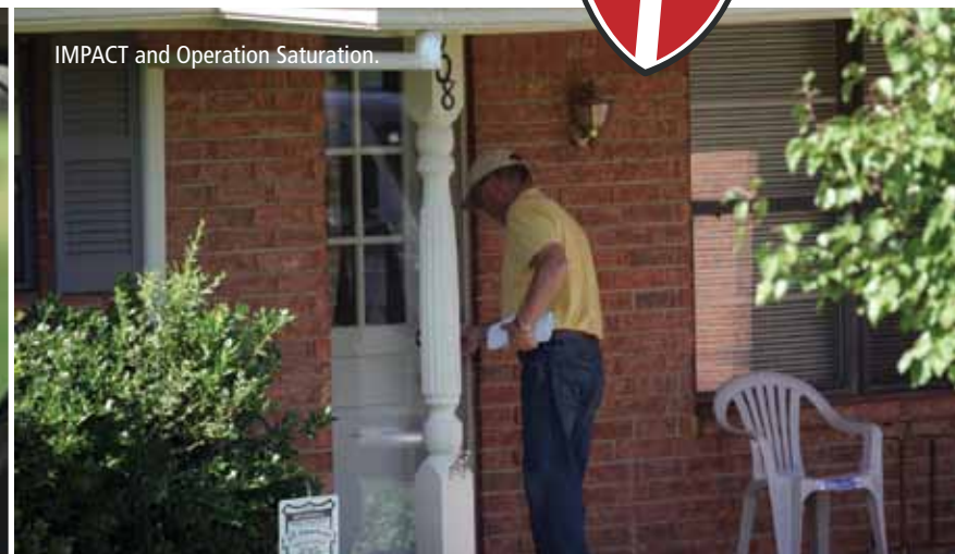
IMPACT construction project.
