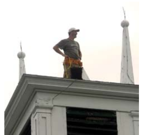
PHOTO (above): Ken Akers surveys reconstruction from atop the belfry.
