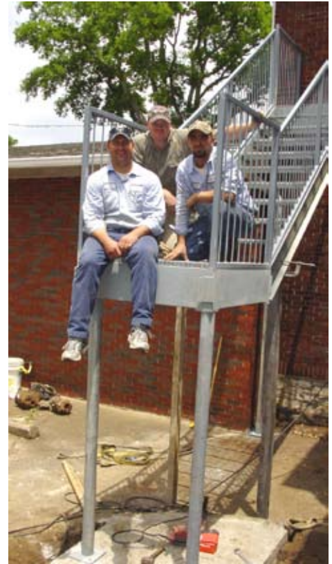
PHOTO IDENTIFICATION: Watch that last step! (L) Mac Atkinson, Jeff Crisp, and Shane Atkinson take a break before attaching the last section to the new emergency exit steps on FWBBC’s Thigpen Building.
